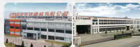
Foshan Shunde - Two Facilities 150000m 2
