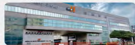
Taiwan Taoyuan Facility 30000m 2
