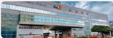
Taiwan Taoyuan Facility 30000m 2
