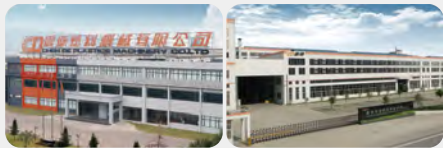
Foshan Shunde - Two Facilities 150000m 2
