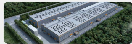
Shanwei Luhe Facility 62360m 2
